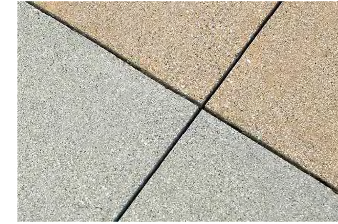
DECORATIVE CONCRETE ACID-ETCH FINISH (WEATHERS' NEW CONCRETE TO EXPOSE FINE AGGREGATES AND ELIMINATE SHEEN AND GLARE OF NEW PLAIN CONCRETE), AS SHOWN OVER PLAIN AND INTEGRALLY COLORED CONCRETE
