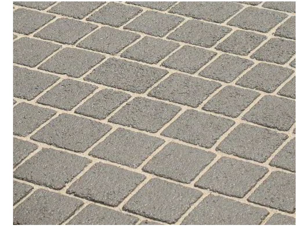
STAMPED ASPHALT (ALTERNATE FOR STAMPED CONCRETE) RANDOM COBBLE, RUNNING BOND (SHOWN WITH STREETBOND COATING WITH CONTRASTING FIELD/GROUT COLORS)
